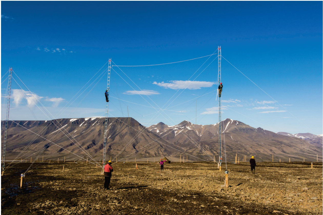
Fig. 2. The SuperDARN radar under construction. Photo: Mikko Syrjäsuo/UNIS.
